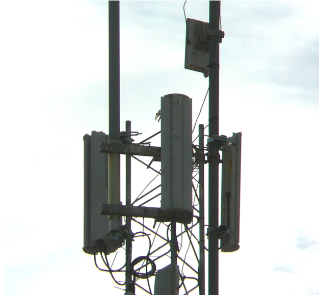
Figure 1: An example of Antelecom's deployment: 3 sector base station (middle) and PTP backhaul (top)
